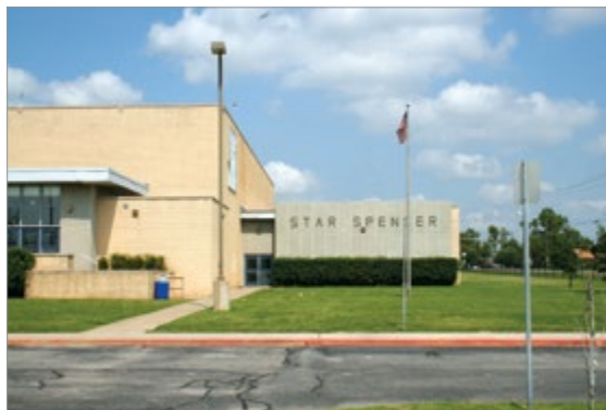
STAR SPENCER HIGH SCHOOL 3001 N. SPENCER ROAD SPENCER, OK 73084 587-8800
